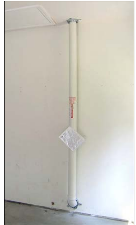
An example of a radon-control vent pipe.
