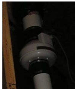
The MDH gold standard requires a full mitigation system to be installed that will not only reduce the radon levels but will reduce the likelihood of other indoor contaminants, that the building code does not consider.
