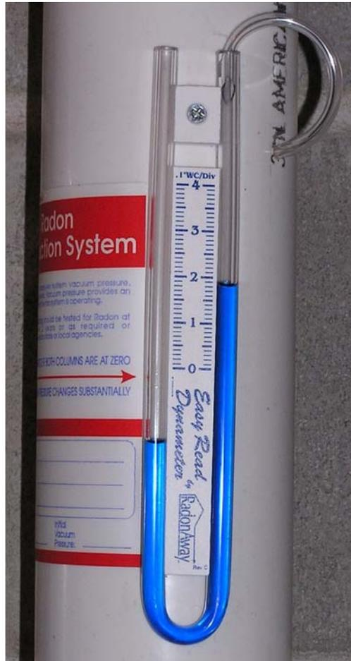
The U-tube manometer is a device to measure pressure differences. A U-tube is a vertical U of bent plastic tubing, the bottom half of which is filled with water. When there is a pressure difference between the two ends of the tube the water is forced to move in the U-tube. This movement is an indication of the changes in pressure. The change or pressure is due to the air being drawn up the radon pipe by the fan.
